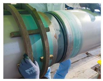
FlexSleeve enables engineers to specify internally-coated carbon steel pipe with welded joints (butt weld or bell & spigot), which is often preferable for many applications.
