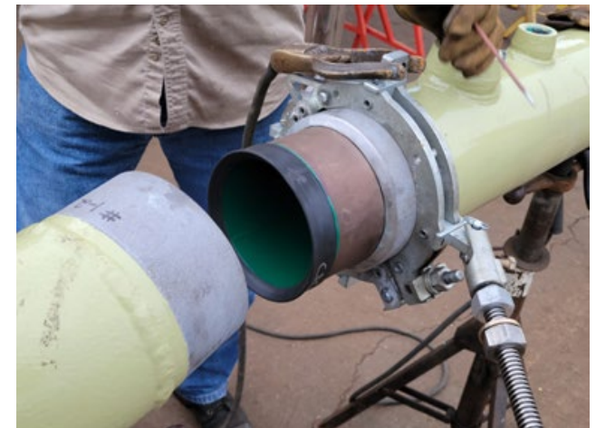
Successful trial installation for offshore service January 2022
