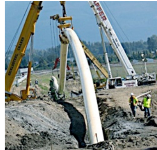
Pipe pulled back during HDD operation. Polyurethane linings & coatings flex with the pipe and have no risk of cracking like epoxy.
