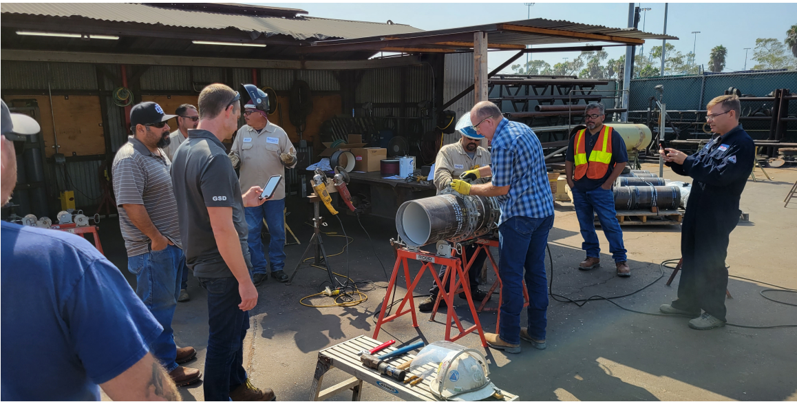
Photos from welding test performed by client prior to approving FlexSleeve for use in a produced water line. FlexSleeve was selected after a side by side test comparison with competitor sleeves. 12" sch. 40 pipe was used for the tests.
