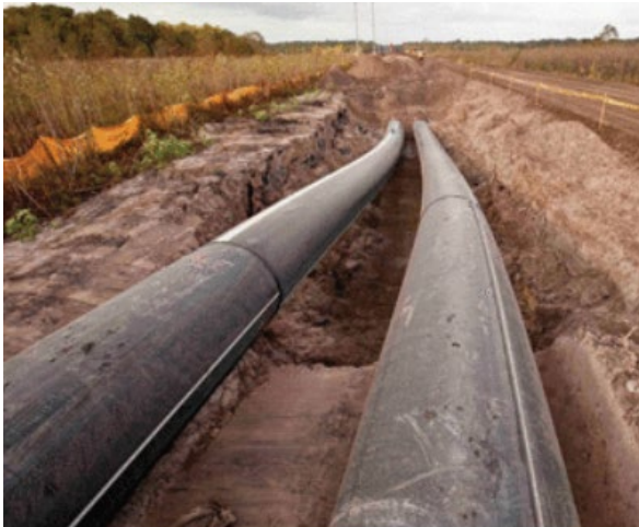
HDPE pipe is widely used for low pressure applications.
